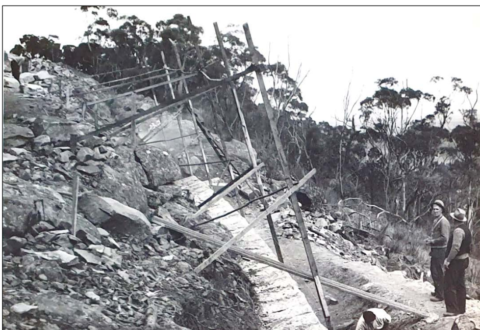
Trachyte retaining wall being built on Mt Gibraltar's north side in 1937 by the Harvey Brothers (Jim at left and Bill). Photo: Paul Harvey. Story on pages 6-7.
