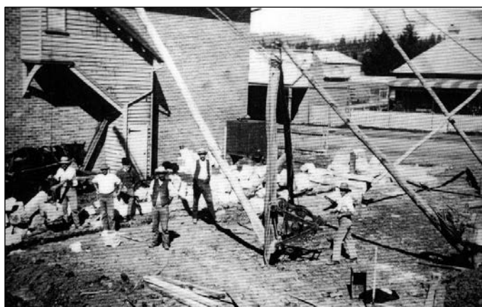
The Hall under construction in 1911
