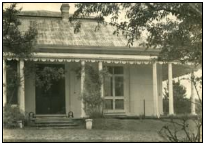
THROSBY HOUSE: Before restoration in the 1970s.
